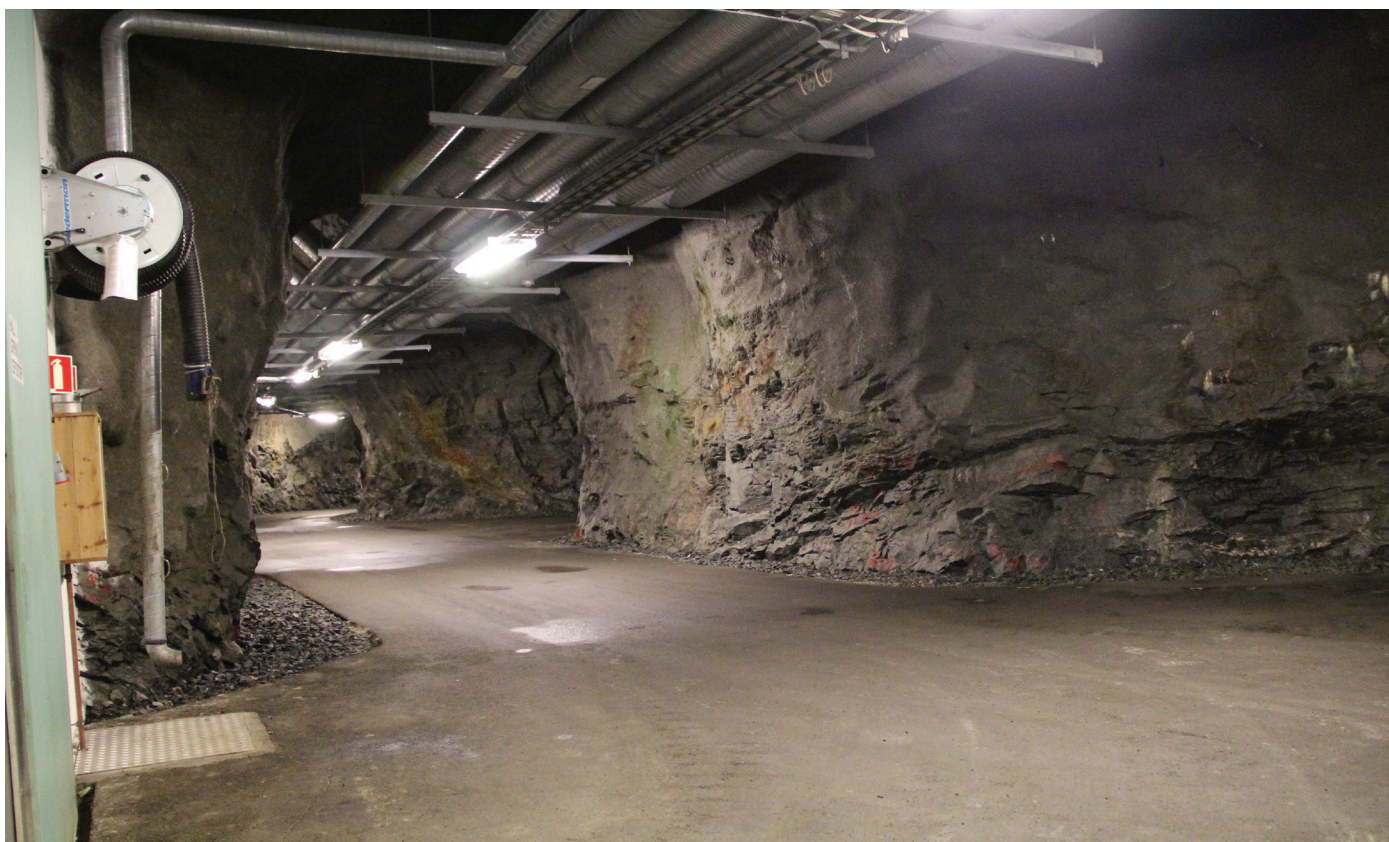
Underground RW disposal facility (Himdalen, Norway)
