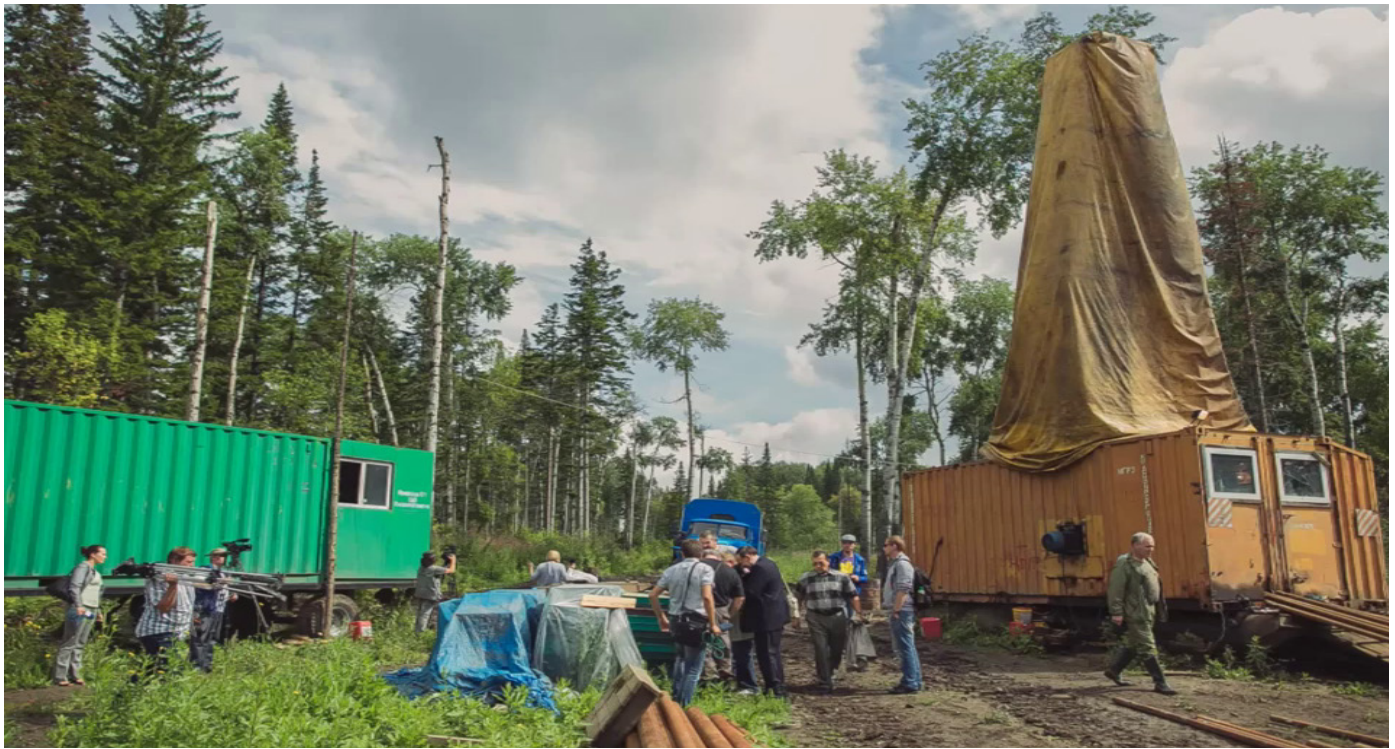
Site for future underground research laboratory
