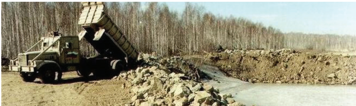
Filling of the Lake of Karachay, storage of medium-level radioactive waste (Mayak plant, closed administrative-territorial unit of Ozersk, Chelyabinsk region)
