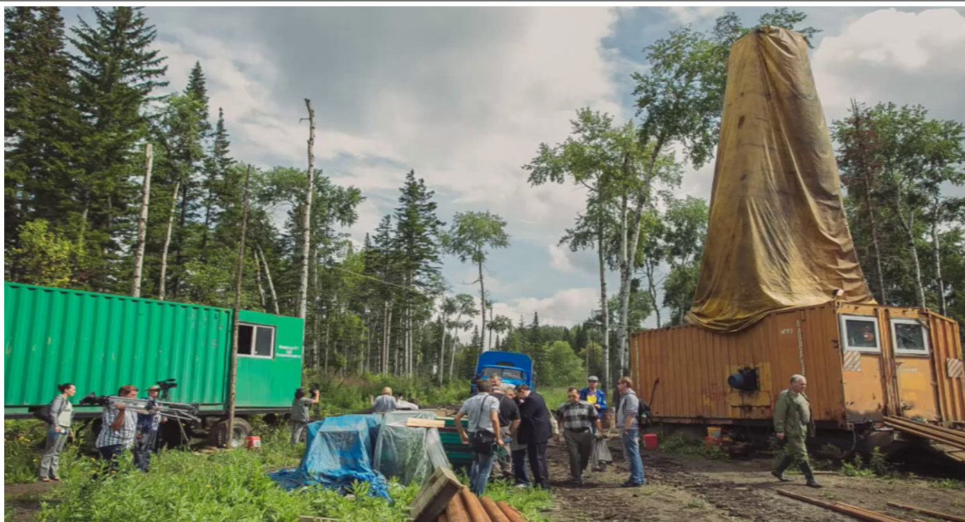
Site for future underground research laboratory
