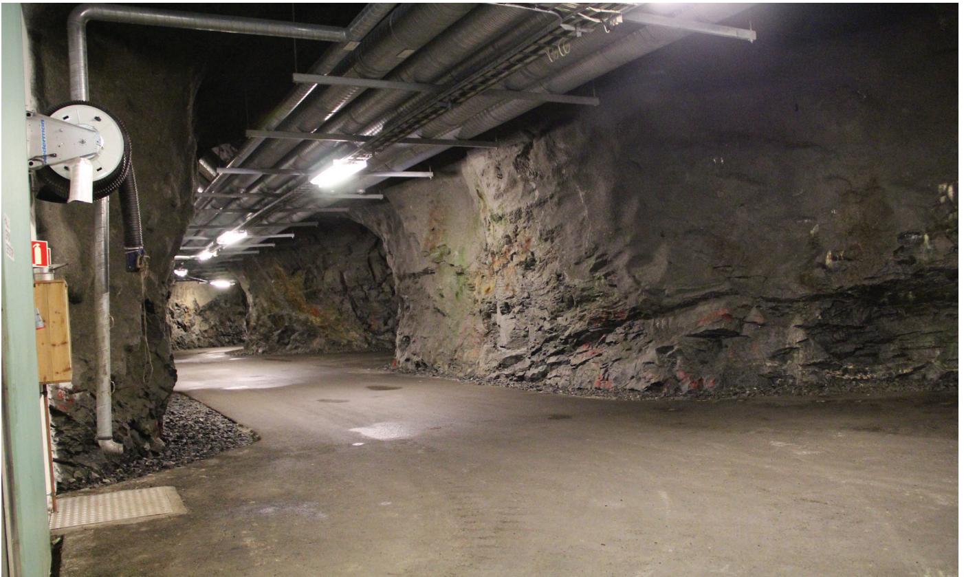
Underground RW disposal facility (Himdalen, Norway)
