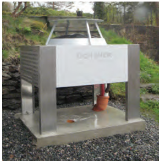
Varmepumpens utedel
