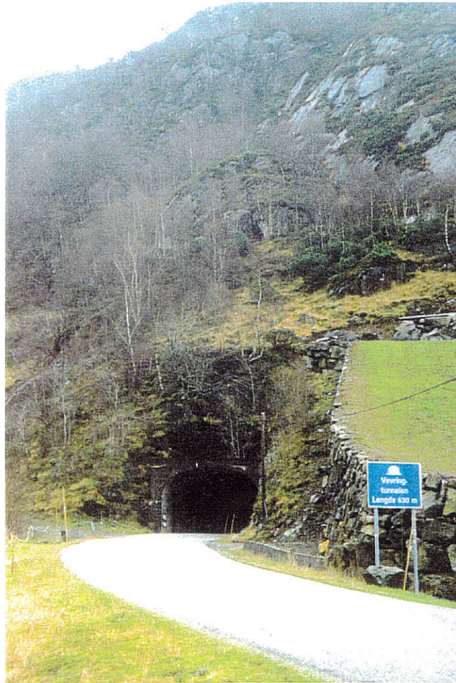
Fig. 2. View of west end of road tunnel through Engebøfjellet
