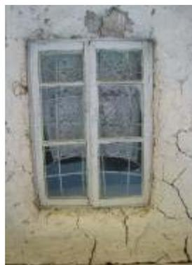
classrooms; window frames had slits and window panes were broken in several places. Besides, there was no water drain (trough) to evacuate water from the roof. In the absence of a socle the back wall of the school building would get wet up to 1.5 from the ground..
